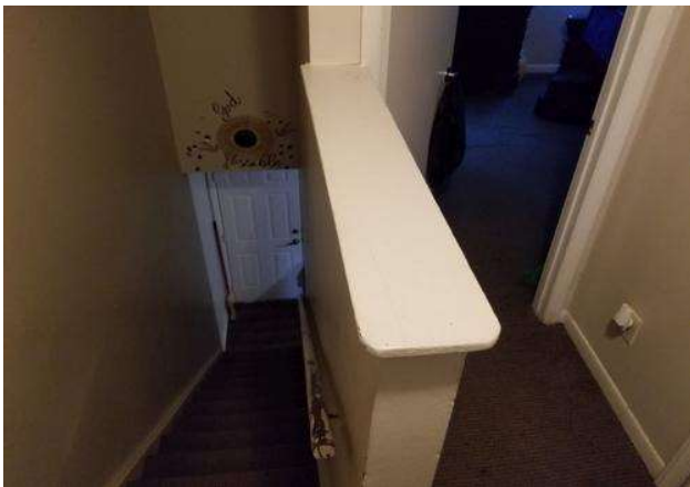
Typical in-unit stairway/walkway
